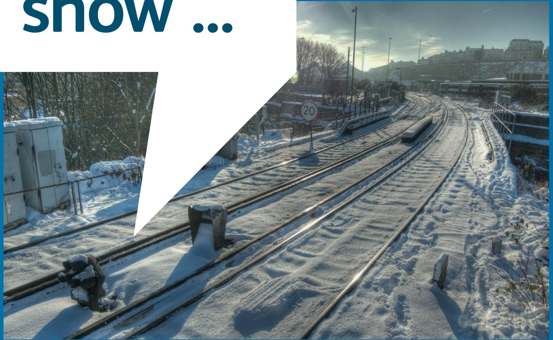
In fact, snow and ice can coat the electrified third rail and overhead lines, preventing your train from drawing the power it
