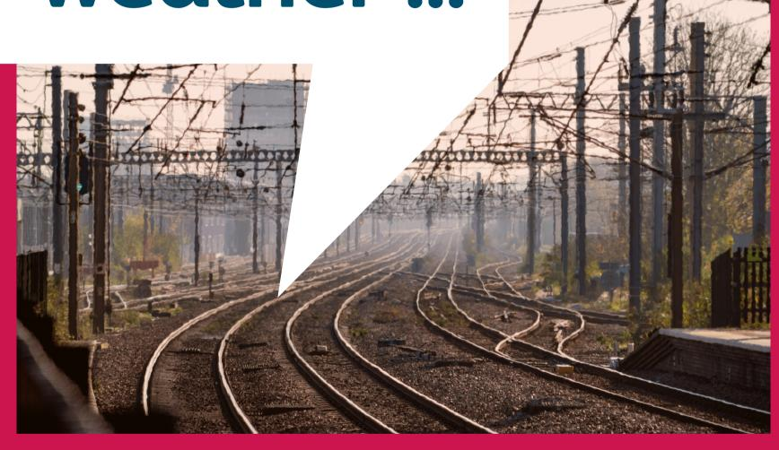
In fact, hot weather can cause the overhead lines to expand and sag. To avoid damaging the lines, trains must travel more slowly than normal.
