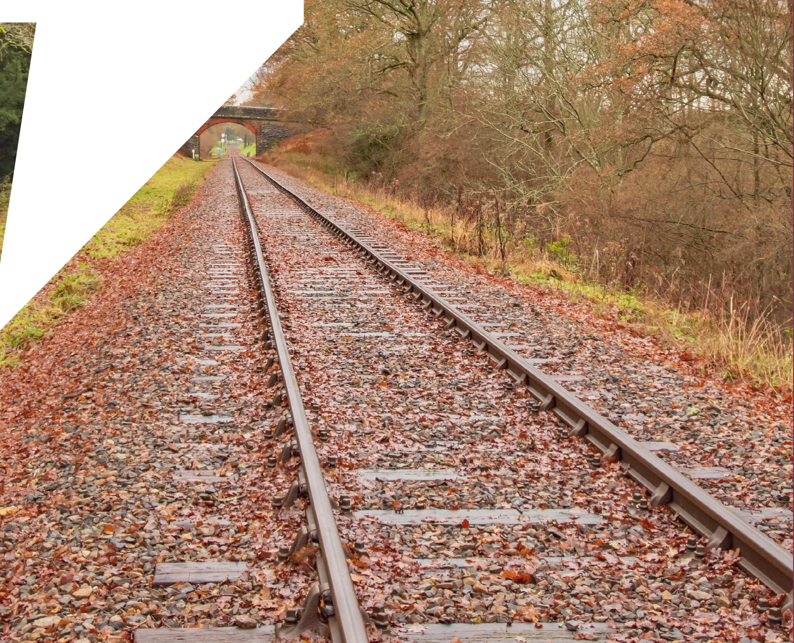
In fact, a build-up of leaves is more likely to stick to the rails. The heat and weight of trains passing over the leaves bakes them into a slippery layer.
