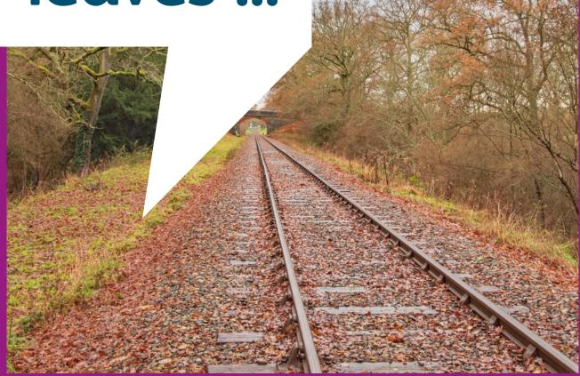
In fact, a build-up of leaves is more likely to stick to the rails. The heat and weight of trains passing over the leaves bakes them into a slippery layer.
